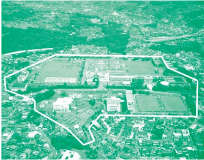
Nishiya Purification Plant
